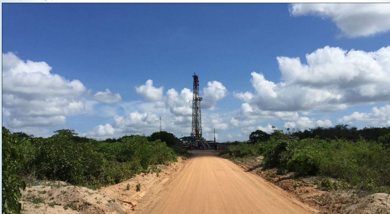
◆ Ntorya-2 drilling operations
