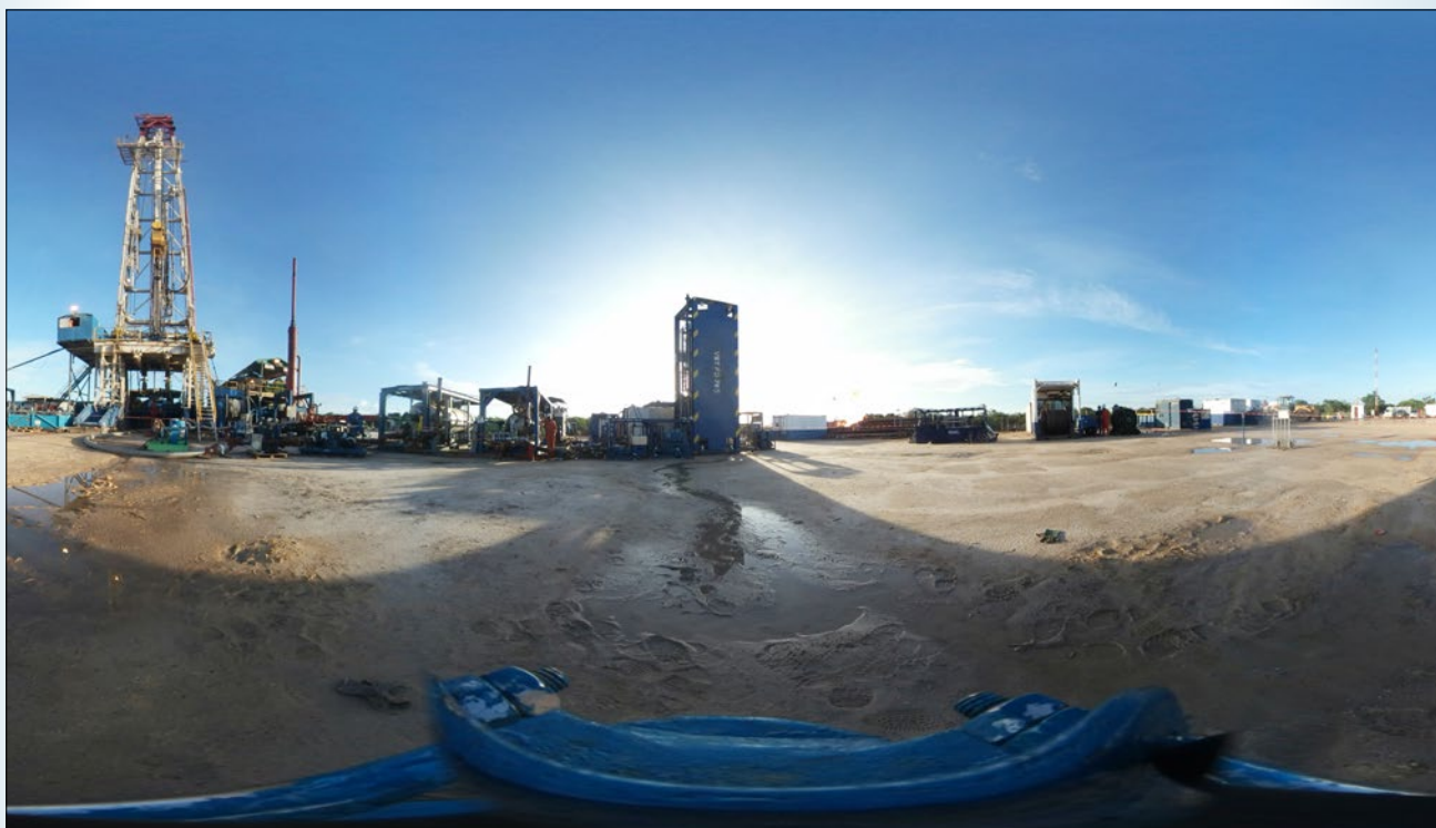
◆ Ntorya-2 drilling operations
