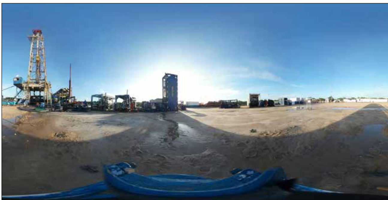
◆ Ntorya-2 drilling operations
