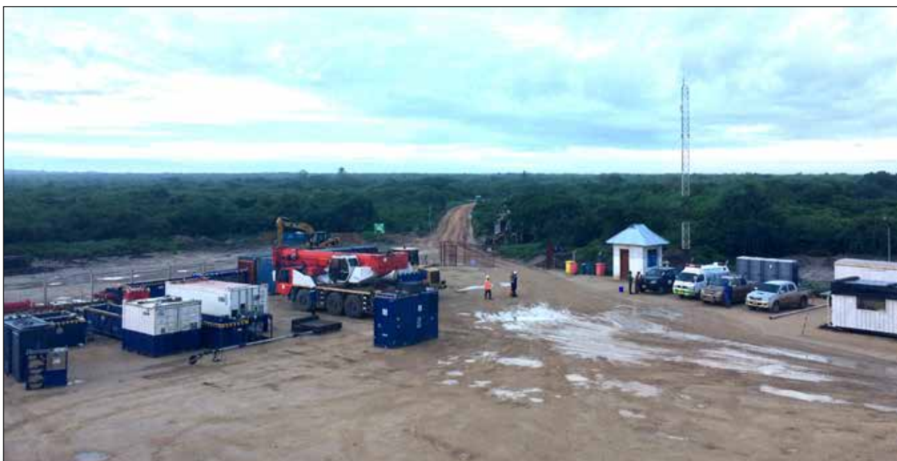
◆ Ntorya-2 drilling operations
