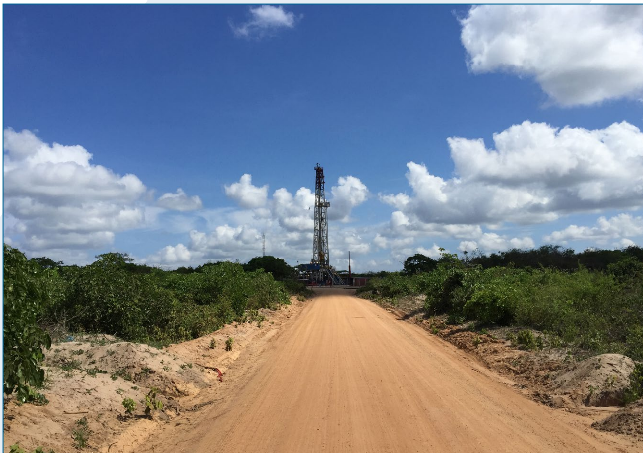
◆ Ntorya-2 drilling operations
