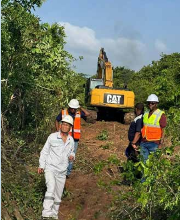
Site clearing commences on Ntorya to Madimba pipeline route
